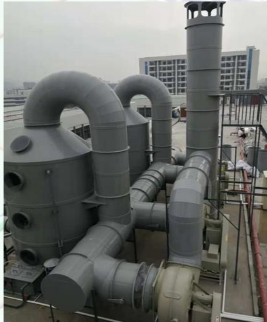
Nickel-Containing Treatment Cap. 40Ton/Hr (Shantou-Guangdong)
